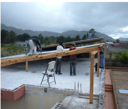
Building our new roof
