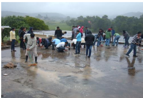
Roof repair—in the rain!
