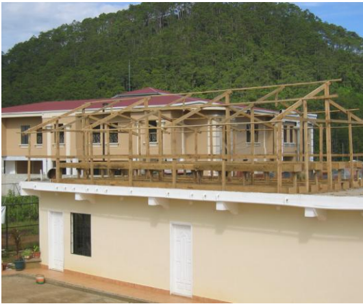
Construction begins on our roof (new Supreme Court building in background)
